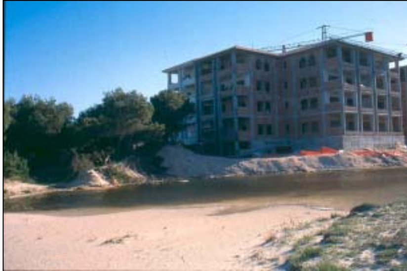
Fig. 5: Construction of a Hotel over the sand dunes field near "S'Oberta".
