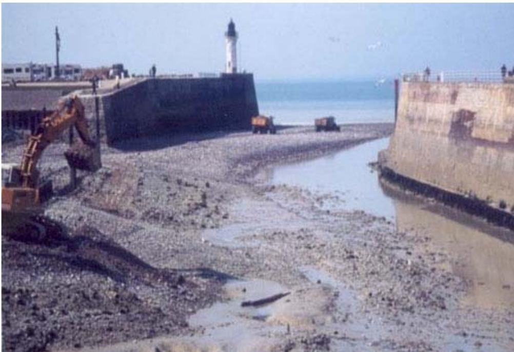
*Fig.12a & 12b: Hard protection on photo A (Pourville) and soft (B) (extraction of the pebble on the harbour and put it on the beaches (Saint-Valéry en Caux)).*
