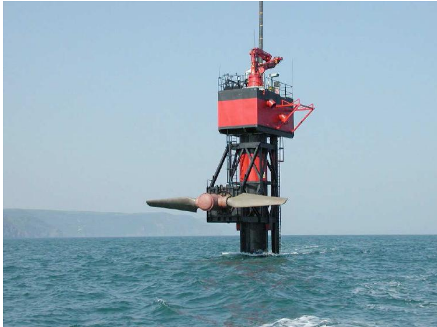
300 kW prototype marine turbine (here the cradle is shown before being submerged in the current)
