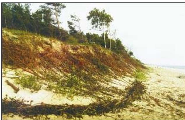
*Fig. 6: Eroded foredune fastened with fences and fascines in Pajuris regional park. Photo: E. Paplauskis, June 2001.*
